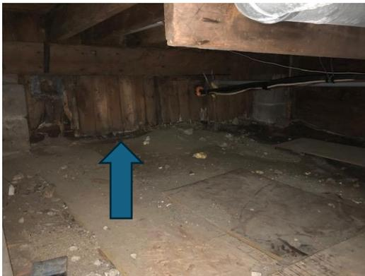
*M: water seepage was noted through the base of west wall in the rear crawl space (wood skirting). The base of the wood skirting should be cut back on the west and south sides, and a concrete curb installed to eliminate any wood/soil contact, and to minimize the risk of leakage into the crawl space. Ensure that water drains away from the wood skirting on the exterior side. Water that gets into the crawl space presently drains below the soil and does not appear to impact the basement area.*
