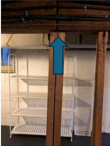
*P: the wood framed wall in the middle of the basement supports two ends of the centre beam. One end needs to be re-supported on a proper steel post. A 2<sup>nd</sup> post is also needed near the furnace. It may be necessary to have proper concrete footings installed below the steel posts.*
