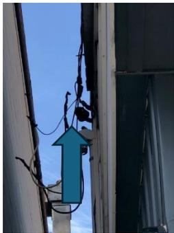
*G: the electrical connections between the incoming service wires and the wires at the top of the electrical mast require proper connectors.*
